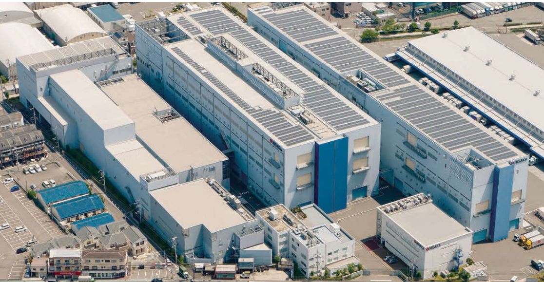
HISAKA WORKS / Konoike Plant
