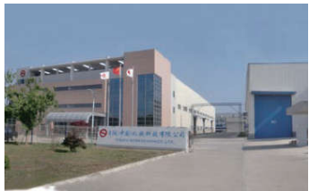
HISAKA WORKS (CHINA) CO., LTD. (China)
